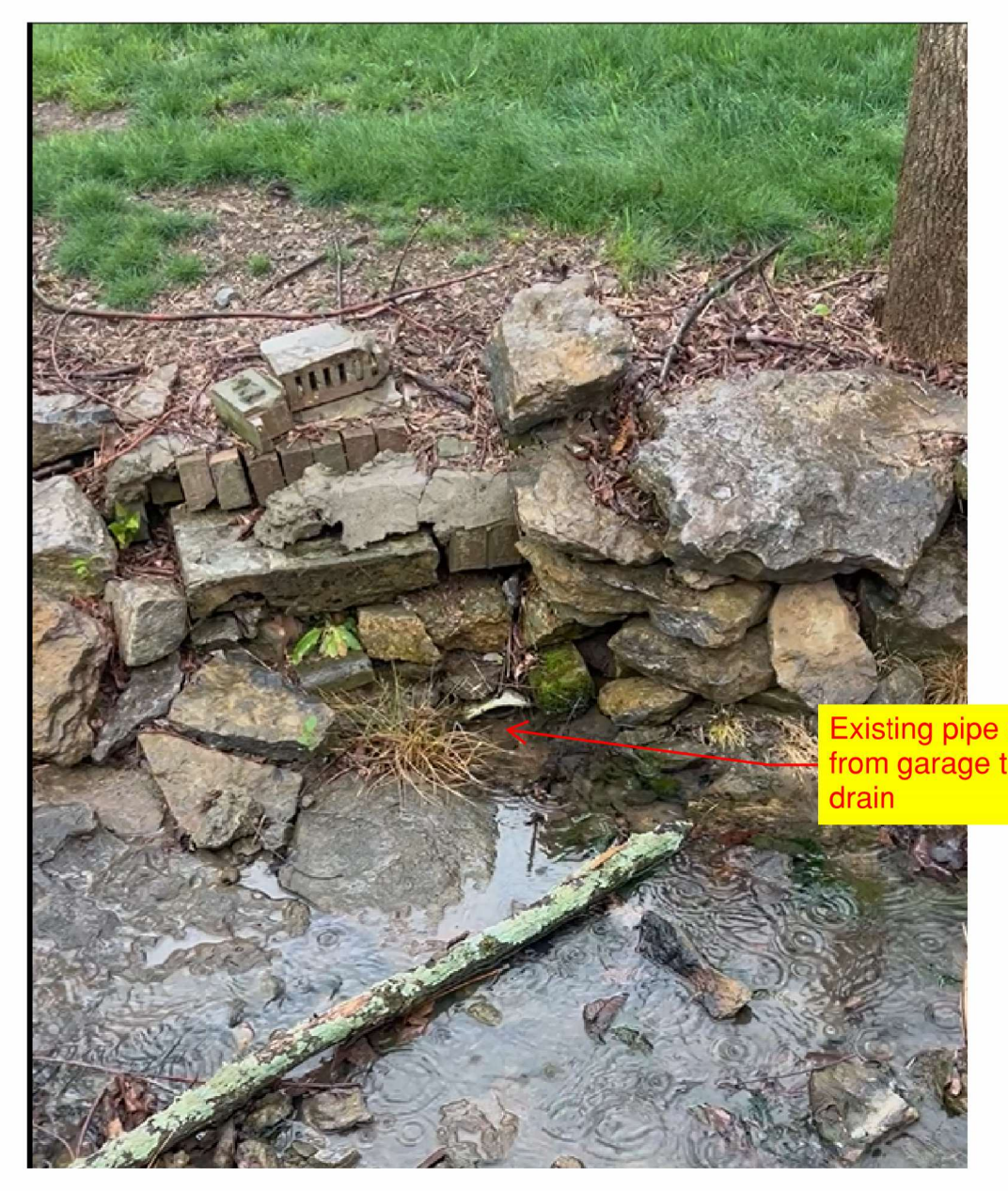
Existing Pipe Outfall
