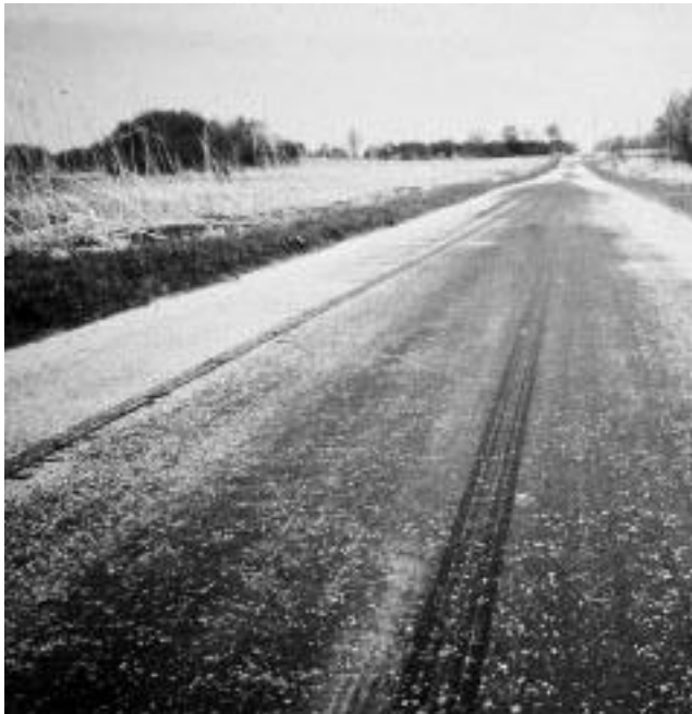
▼ Severe flushing.
