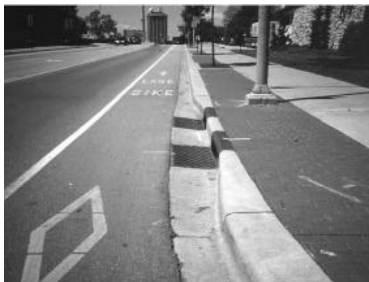
Urban drainage. RATING: Excellent
