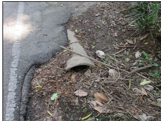
Figure 3: Existing Storm Drainage Pipes
