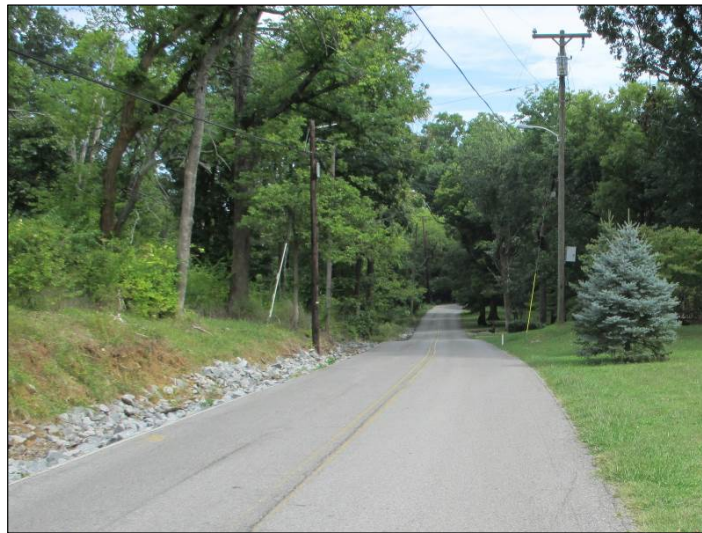
Figure 4: Existing Overhead Utility Lines
