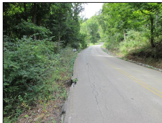
Figure 5: Existing Pavement Surface with Cracking
