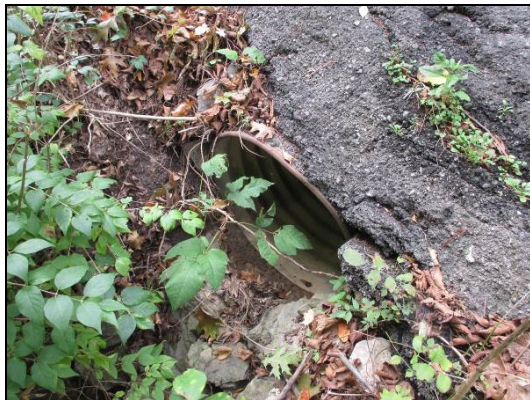
Figure 3: Existing Storm Drainage Pipes
