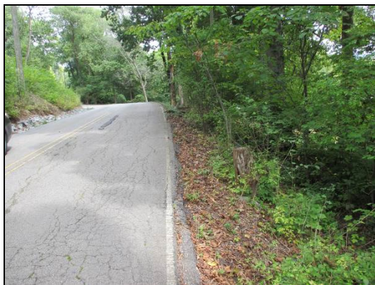
Figure 5: Existing Pavement Surface with Cracking
