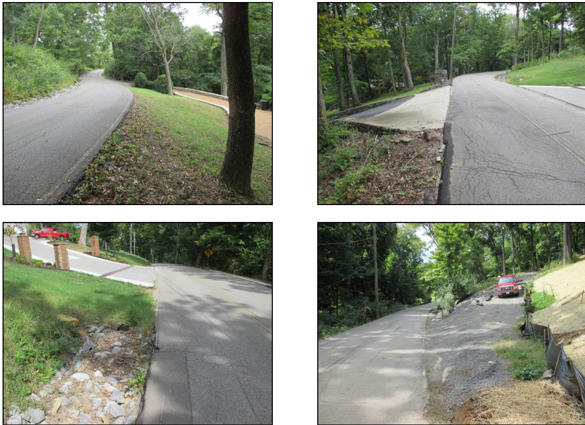
Figure 13: Existing Driveways that will Require Special Consideration if Widened
